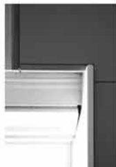
Detail view of refurbished ash window and new wainscoting with walnut capping
