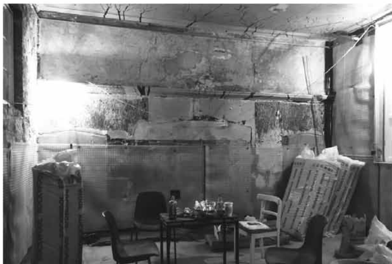
Damp Proofing: Installation of new Delta membrane up to 1.2m throughout and full-height to front external wall and in Room 9.
