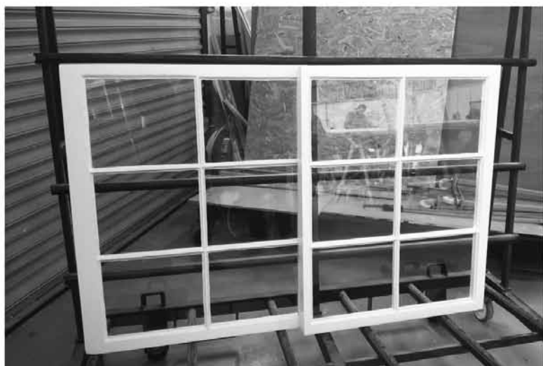
Wooden structures removal, fitting and painting: Removal, restoration and painting of original timber, single-glazed, sliding-sash windows.
