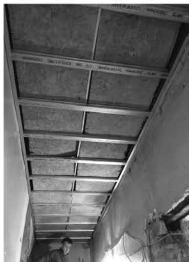
Ceiling finishes: Installation of new 60-minute fire-rated ceiling to underside of original ceiling. Structure and insulation (left) and finishes plasterboard (right).
