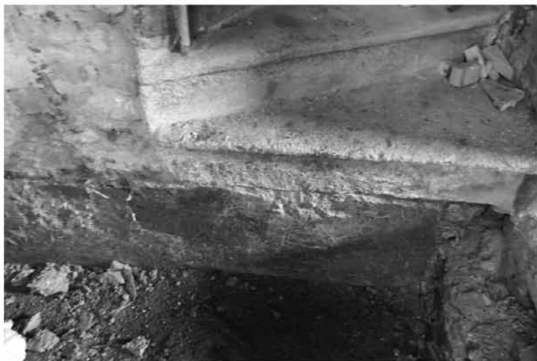
Internal walls structure: Underpinning structural works to internal original granite stairs.
