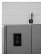
Detail view of new wainscoting, new switch panel and new ironmongery.
