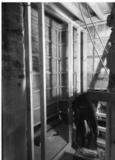
Internal walls: Studwork for new internal walls. Boxing out to allow for ducting behind finished wall.
