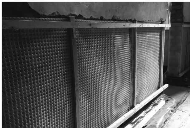
Internal walls: Boxing out to internal walls to allow for ducting behind finished wall panelling, to dado rail height.
