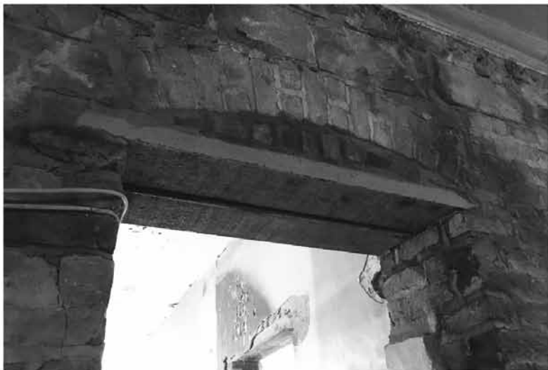
Internal walls structure: Removal of original, rotten, timber lintels where failing and installation of new concrete lintels. Stitching and filling of cracks where necessary (top right of photo).
