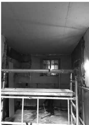
Ceiling finishes: Installation of new 60-minute fire-rated ceiling to underside of original ceiling. Structure and insulation (left) and finishes plasterboard (right).
