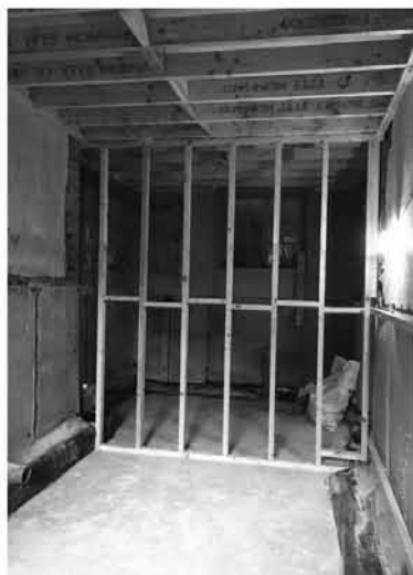
Internal walls: Studwork for new internal walls. Boxing out to allow for ducting behind finished wall.
