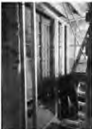
Internal wall structure for new internal walls. Bracing stud for window to cladding behind (cladding wall).
