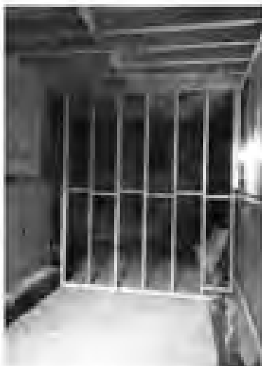
Internal wall structure for new internal walls. Bracing stud for window to cladding behind (cladding wall).
