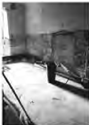
Demolition and Alterations: Pouring of new floor slab with DPM (dimpled plastic membrane) installed. Blasting up and venting of existing fireplace and masonry openings.
