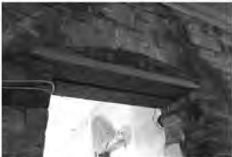
Internal walls structures. Removal of original, rotten, broken timbers where falling and installation of new concrete timbers. Skirting and filling of cracks where necessary (top right of photo).
