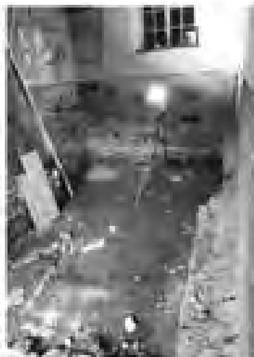
Demolition and Alterations: Chopping out old existing floor slab. Removal of existing wall finishes: Removal of existing lime plaster up to 1.0m everywhere (left) and full-height on front external wall (right).
