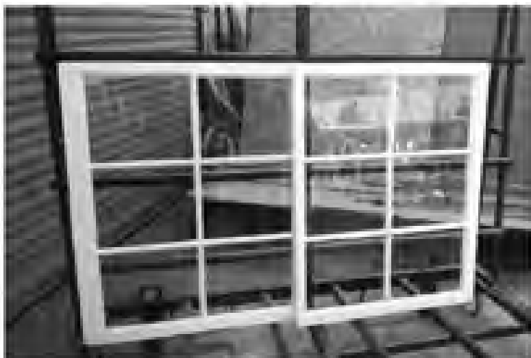
Wooden structures removed, fitting and painting. Removal, restoration and painting of original timber, single glazed, sliding patio windows.
