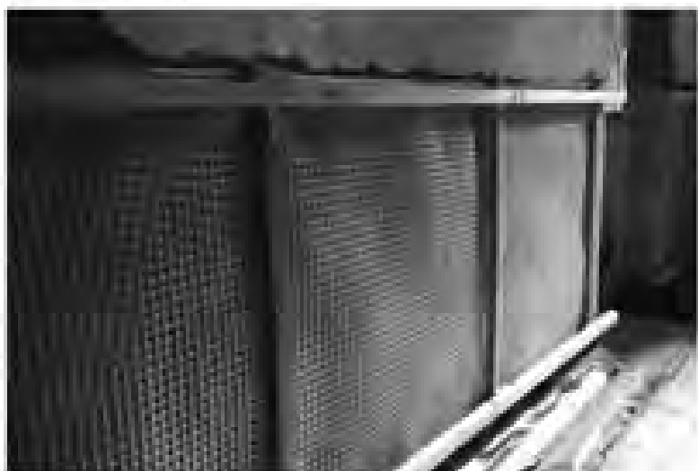
Internal walls: lining out to internal walls to allow for ducting behind finished wall paneling, to ducts wall fixtures.
